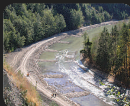
RIVER FLOW IS REINTRODUCED INTO THE ENGINEERED CHANNEL.
